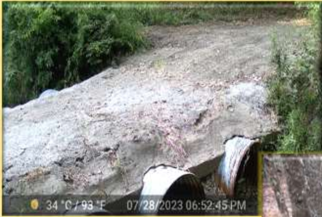
Creek Crossing Repair
